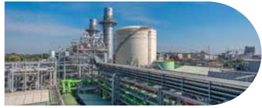
POWER GENERATION AND WATER TREATMENT
