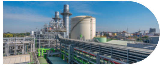
POWER GENERATION AND WATER TREATMENT
